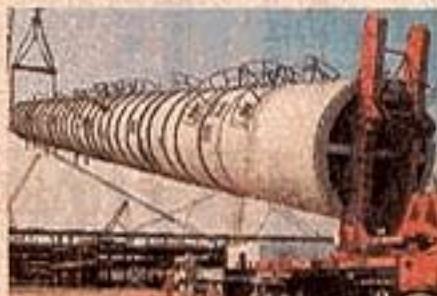
KNM's 100-ton high-pressure pump is being moved by a crane.
